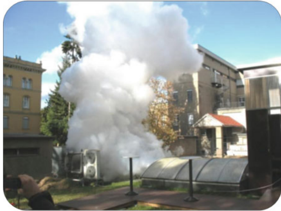
Fig. 7.20 Quench gas release through quench duct after decommissioning a cryomodule for MRI (MRI magnet installed in hospital basement)
